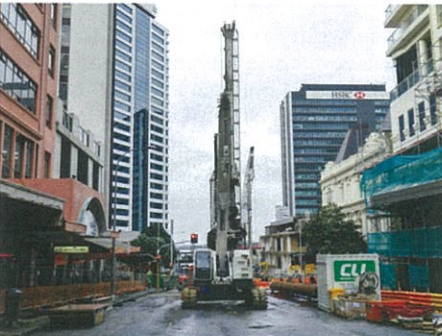
The Soilmec SR100 cased CCFA piling rig is the first ever to be used in New Zealand
