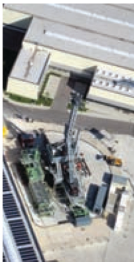
A PR 300/440 M1 drilling a geothermal test well
