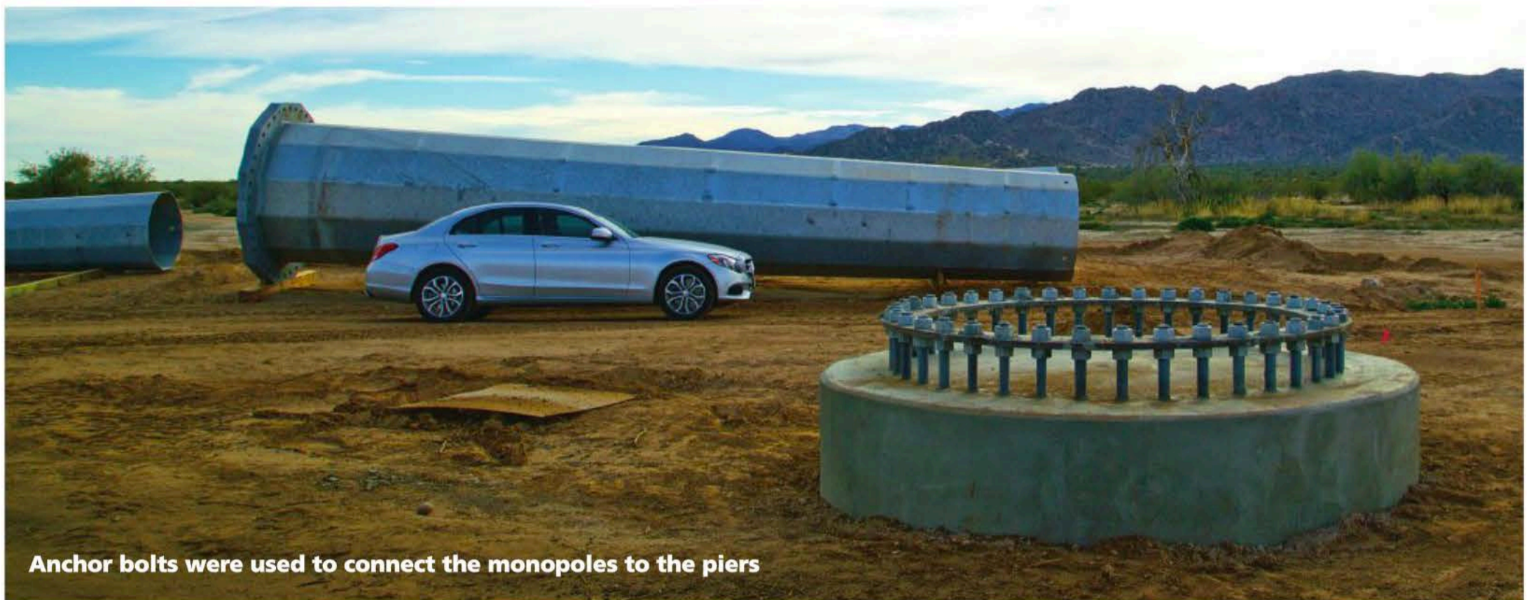
Full-length anchor bolt cages were used to secure the monopoles
