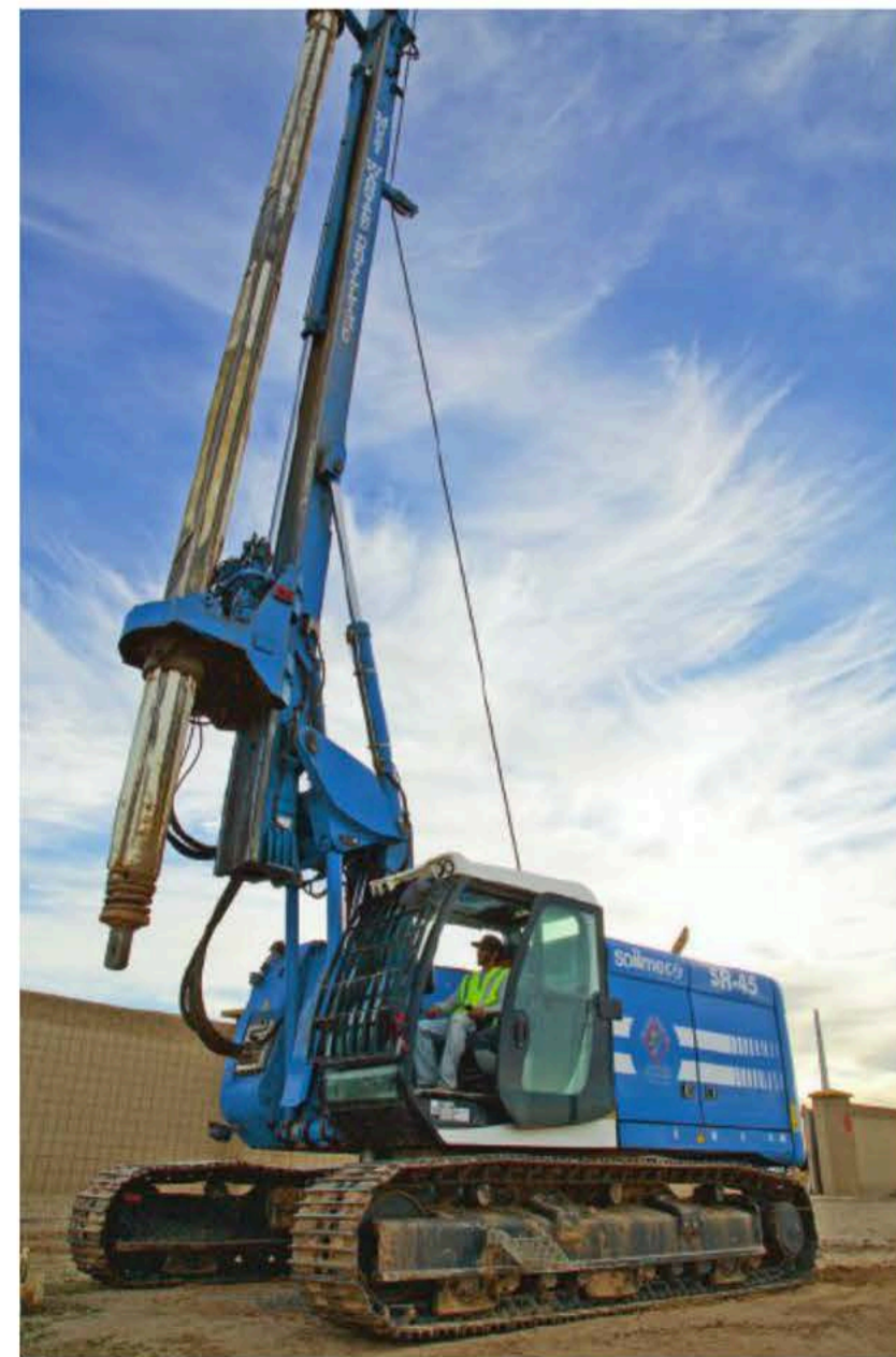
Power line pier foundations were installed with a Soilmec SR-45
