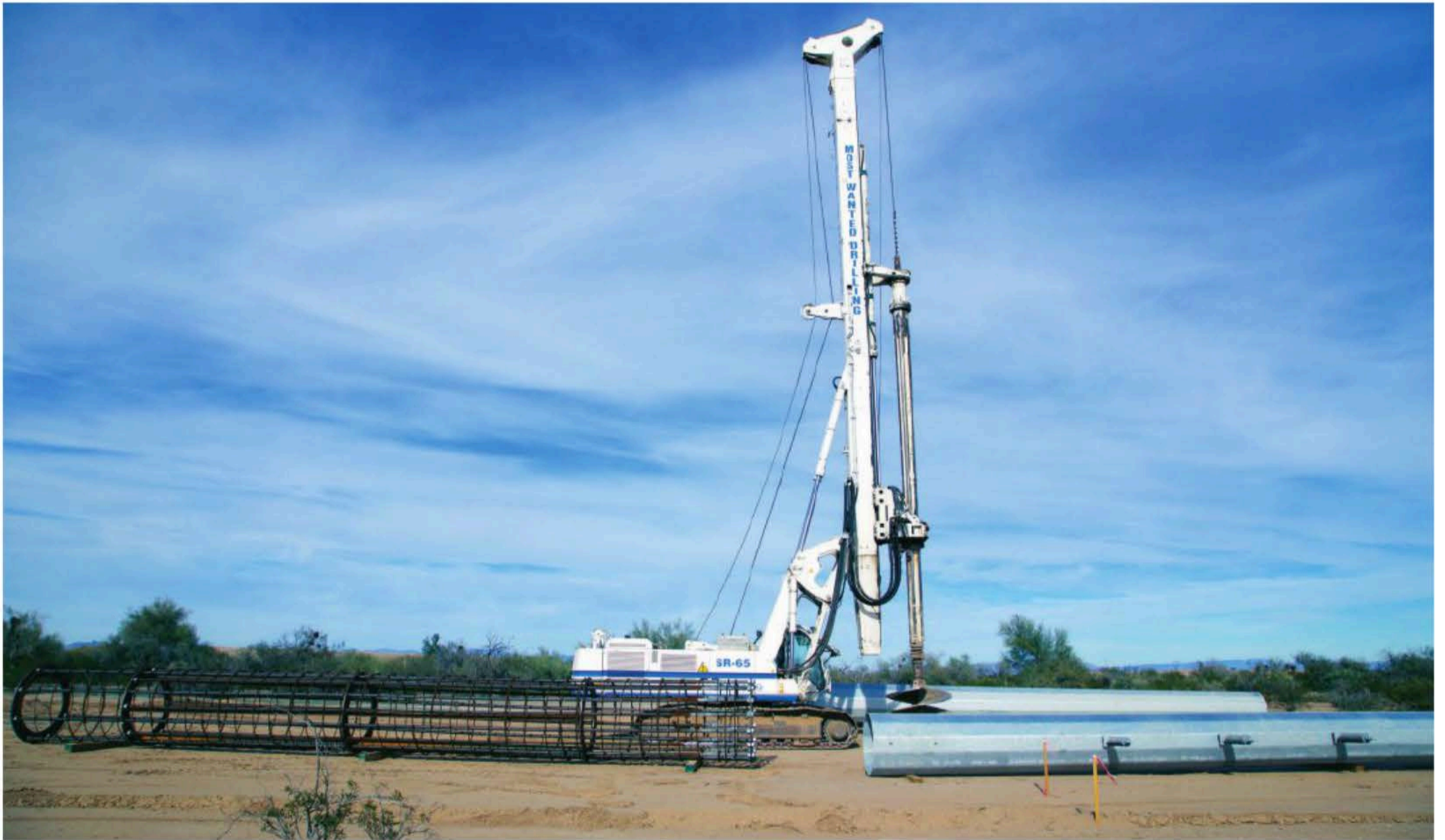
Soilmec SR-65 installing 11 ft (3.3 m) diameter piles
