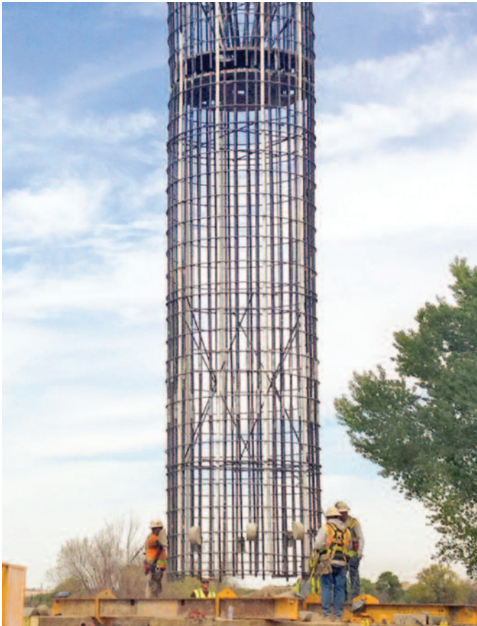
Placement of reinforcing steel for 120-inch-diameter shaft with O-Cell visible.
