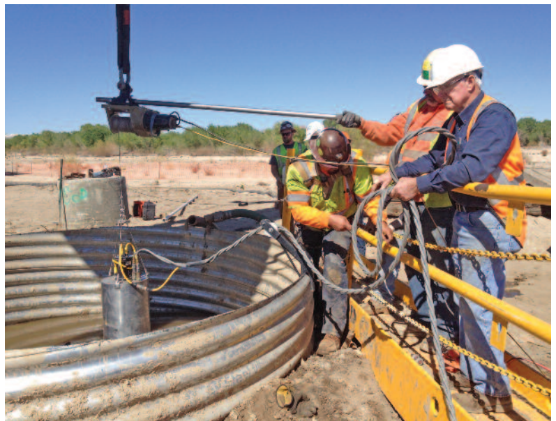
Inspection of 120-inch-diameter shaft with the Mini SID.
