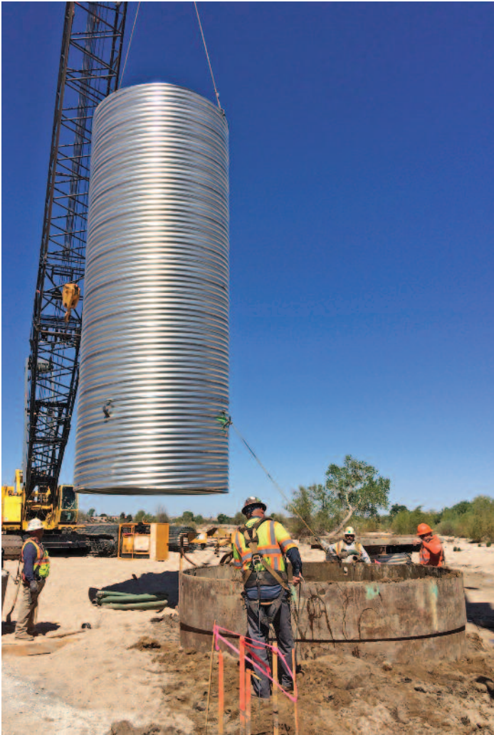
Preparing to lower the corrugated metal pipe into position.
