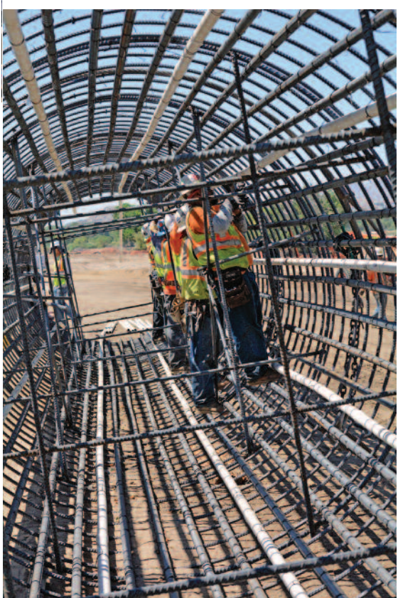
Installing PVC pipes (test tubes) for Gamma-Gamma testing after shaft construction.
