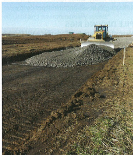
Tensar International provided its TriAx multi-directional geogrid product for the construction of 24km of access road for the Keadby wind farm site
