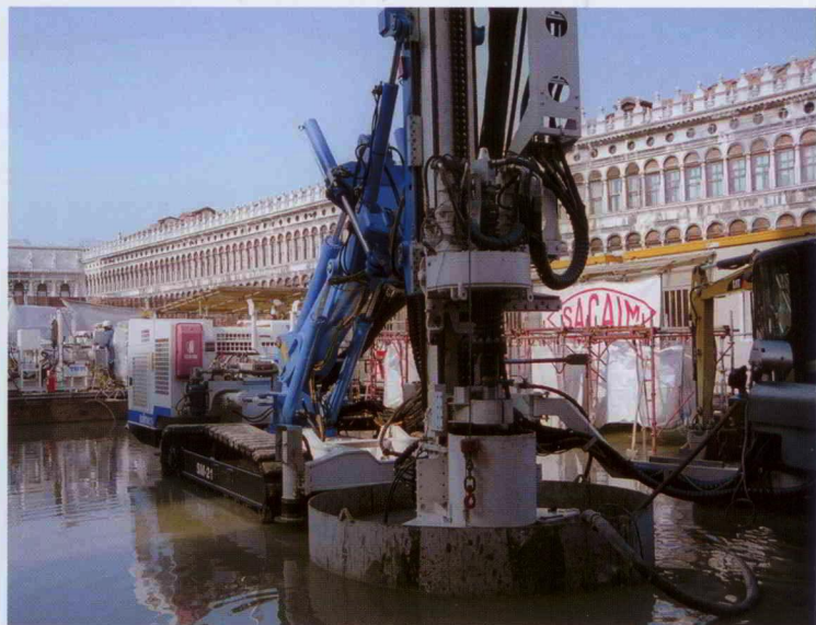
The job site with "acqua alta" (high tide)
