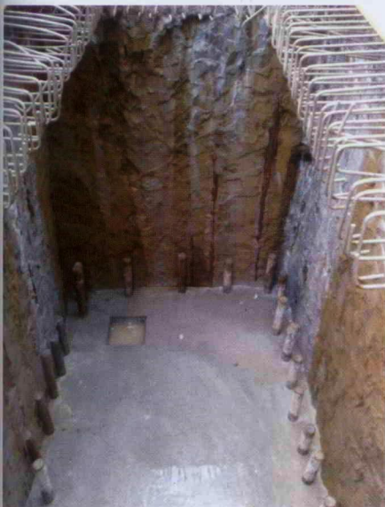
Watertight work pit for deep soil mixing in Venice
