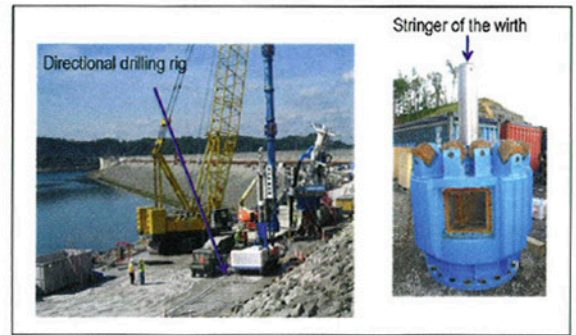
Fig. 6. Directional drilling rig and piles construction.
