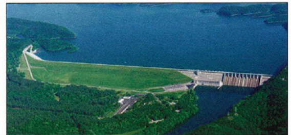
(b) General view of the Wolf Creek dam.
