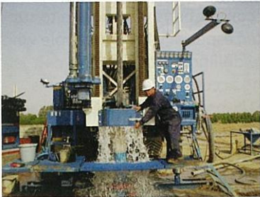
Drillmec Drilling Superintendent on Site
