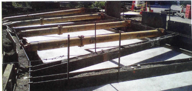
Hydraulic struts in place on shoring.
