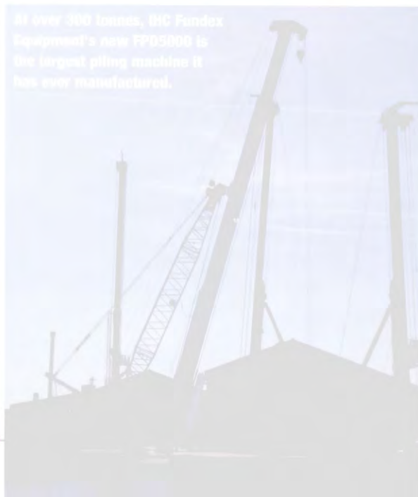
Bachy Soletanche's Heavy Duty Large Diameter Auger rigs are being used to install the piling for four large wind turbines in the UK.
