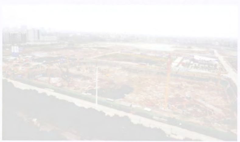
Seven Liebherr SH 855 HD crawler cranes – four HS 855 HDs and three HS 885 HDs (pictured) – have been compacting a ground area of 6.5 km 2 for a new town in Kuwait.
