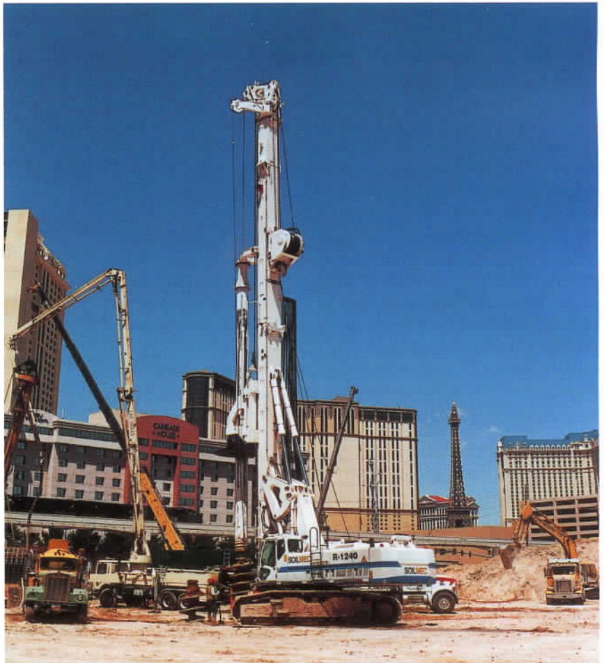
Drilling in Las Vegas, Nevada.
