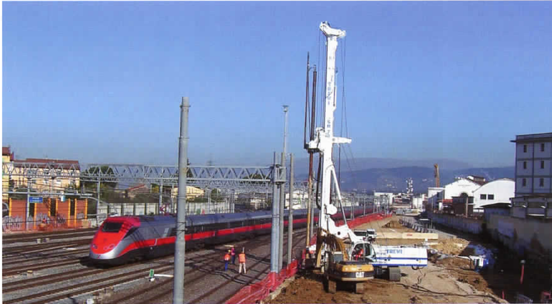
High speed rail station being built in Florence, Italy.
