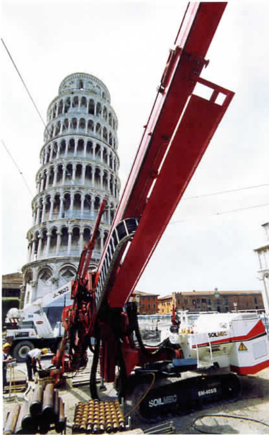
Work under way at iconic tower in Pisa.
