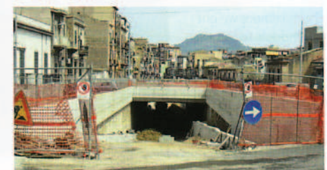
Construction of underground passage
