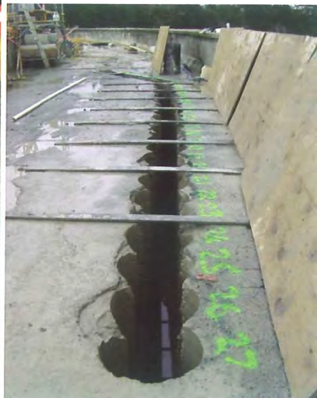
LEFT: Pouring slot for concrete using a tremie pipe. ABOVE: A line of pre-drilled holes five metres deep.
