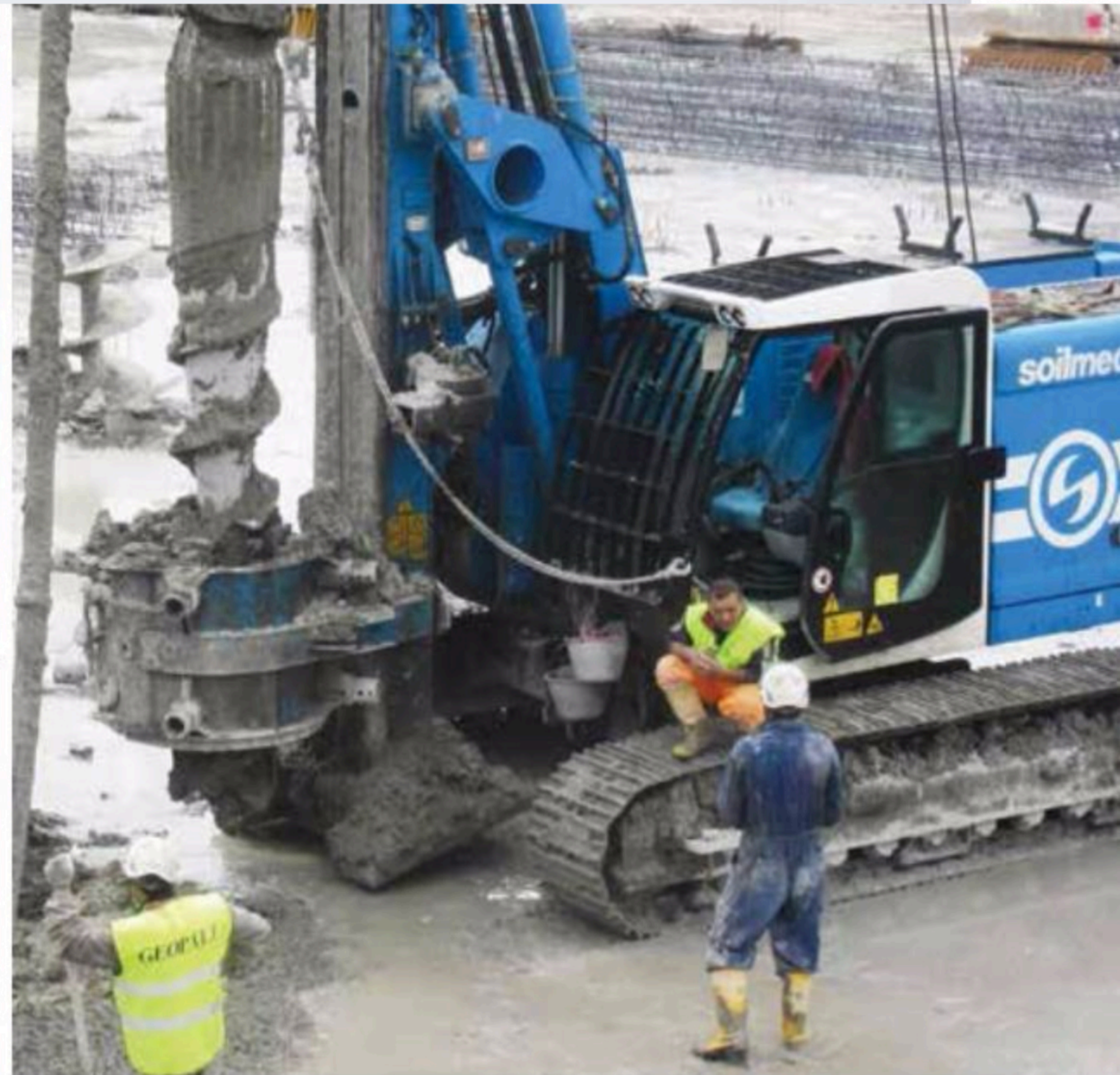
Above: The SR-45 is equipped with the Soilmec DMS system in order to have total control over the rig performance and site production rates.
