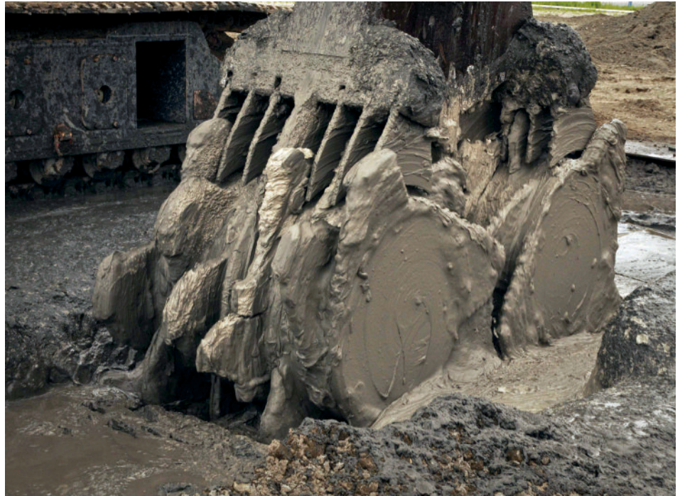
Cutter soil mixing wheels in use (credit, Keller)
