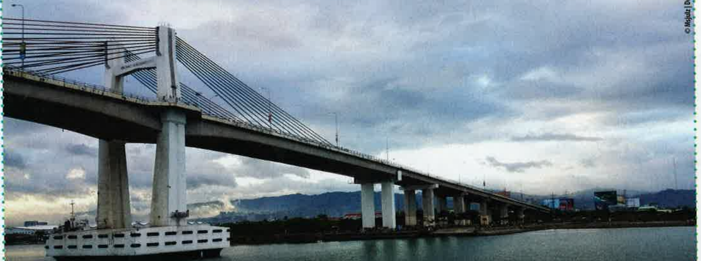
Marcelo Fernan Bridge
