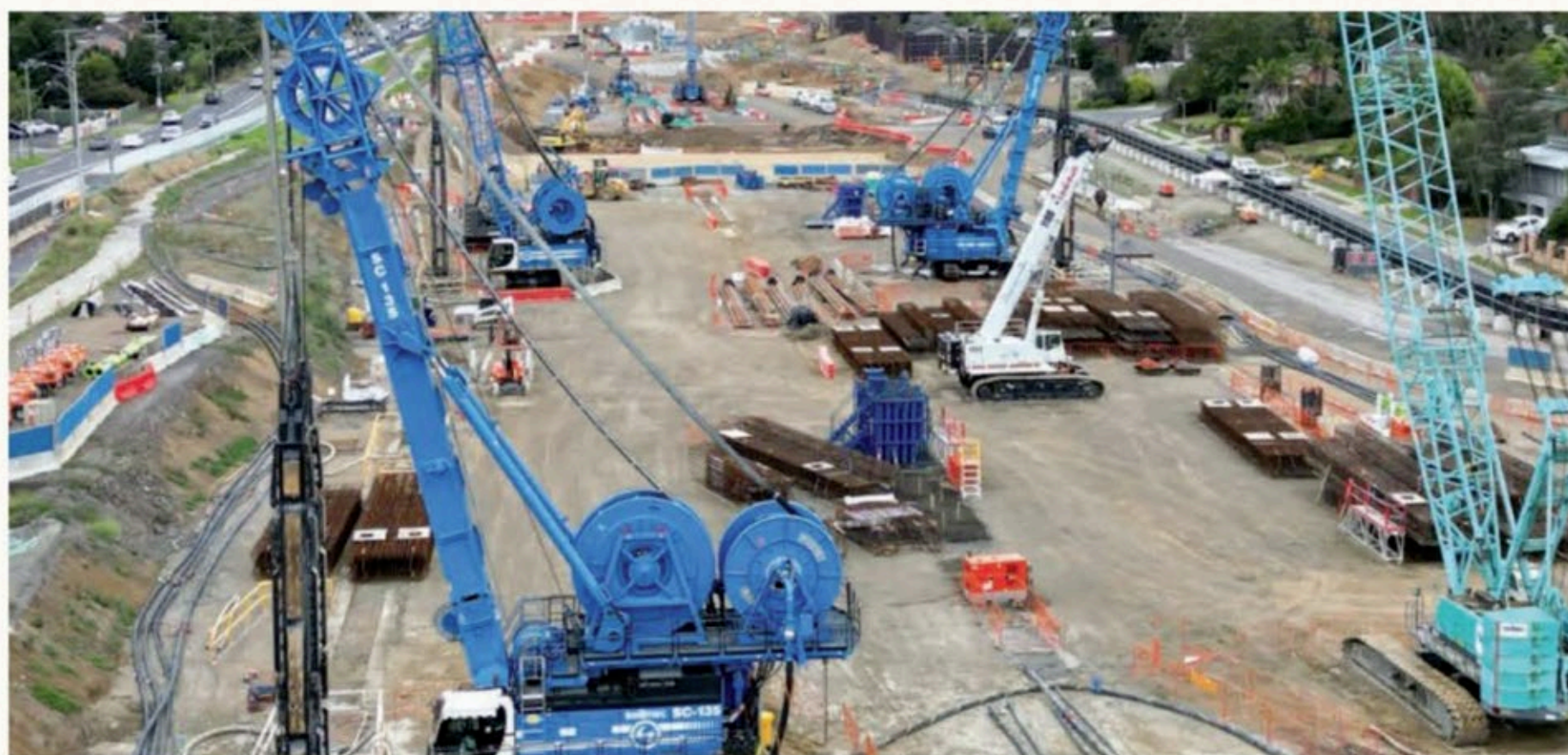
Trevi Group working on the North Link project in Melbourne, Australia
